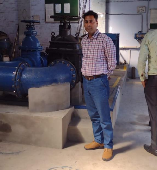
350 mm pipeline with valve to test VT Pumps upto 400 HP
