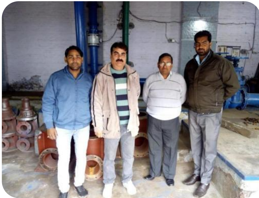
Inspection and testing of pumps done by Shri Kaushal Kumar Prajapati (Asst. Executive Engineer) from Bhakra Beas Management Board (BBMB) Nangal Township Punjab
