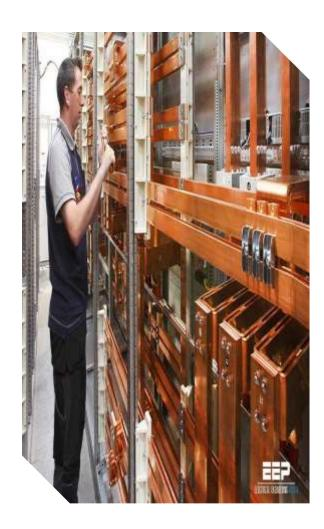
**Total Type Tested Panel**: Upto 4000 Amp / 50 kA for 1 sec Conforms to IEC 61439
